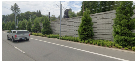
TREATMENT ALONG ROADWAY IMAGE SOURCE: GOOGLE EARTH
