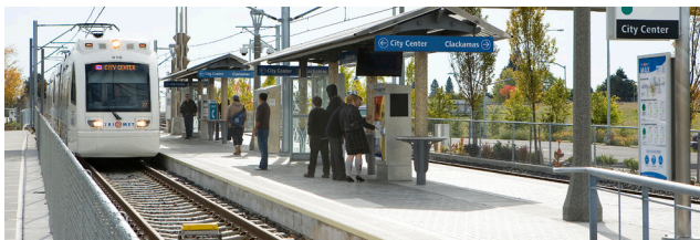
AT-GRADE TRACK IMAGE SOURCE: TRIMET FLICKR
