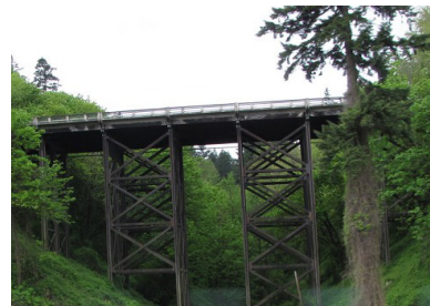
EXISTING VIADUCT IMAGE SOURCE: STRUCTURAE.NET
