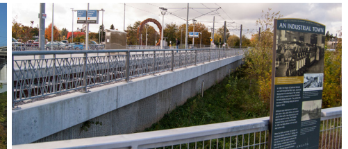
TREATMENT WITH PROTECTIVE RAIL IMAGE SOURCE: DAVID EVANS AND ASSOCIATES
