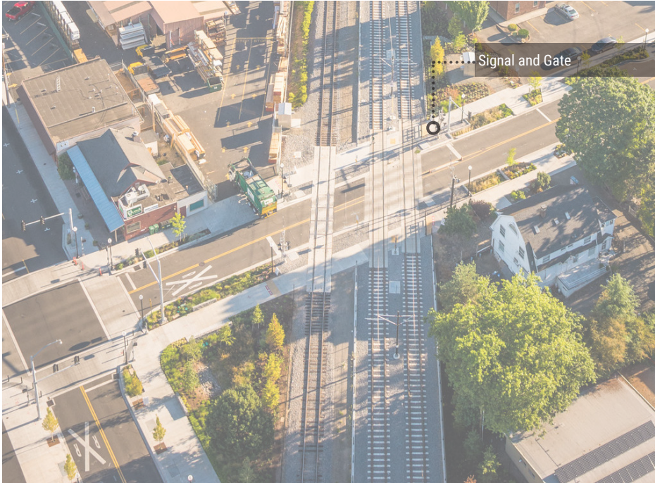
SHARED LIGHT RAIL-RAILROAD INTERSECTION (DOWNTOWN MILWAUKIE)
