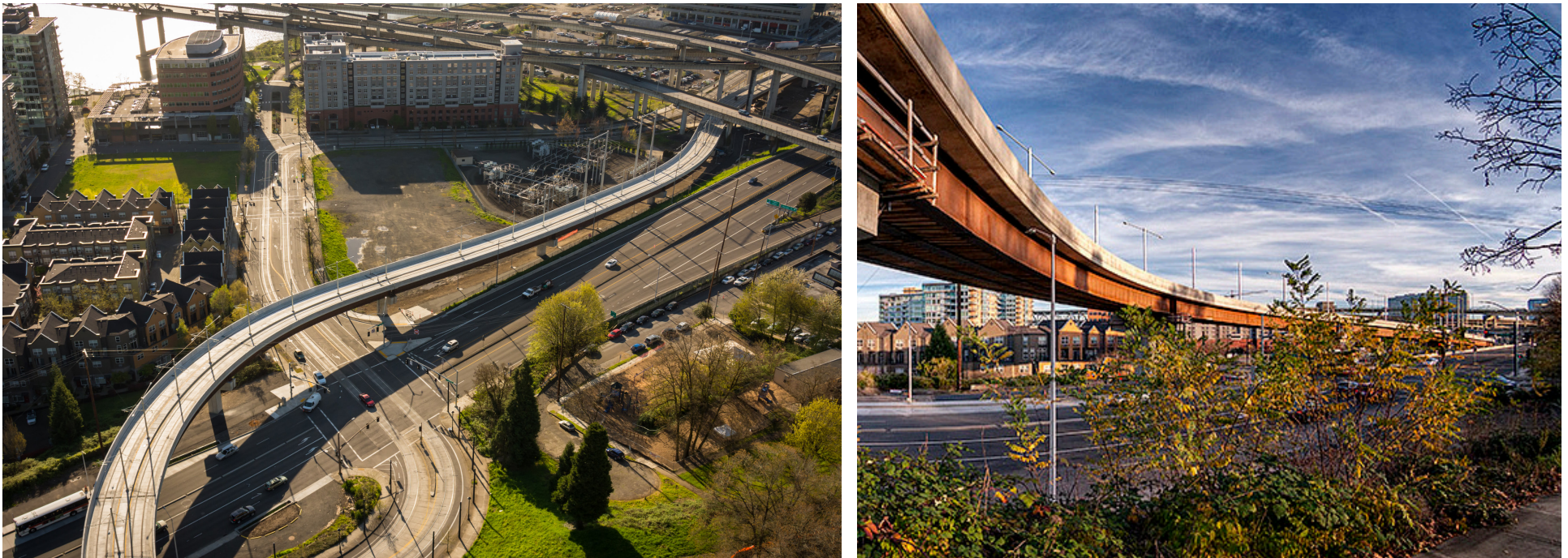
Figure 5.8.4 Bird's eye view of Harbor Structure, which is similar to the viaduct replacements (Image Sources: TriMet Flickr, Victor von Salza Flickr)
