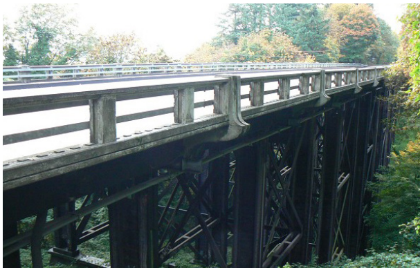
Figure 5.8.2 Vermont Viaduct (Image Source: Structurae)
