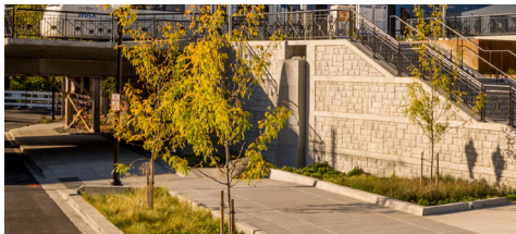
ABUTMENT WALL AND STAIRCASE IMAGE SOURCE: TRIMET FLICKR
