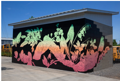
SUBSTATION IMAGE SOURCE: MEG ADAMSON
