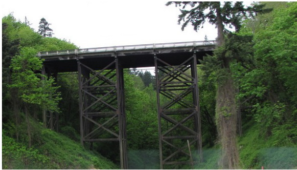
Figure 5.8.1 Newbury Viaduct (Image Source: Structurae)
